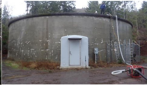
Left: Odell Water Reservoir Right: Booth Hill Reservoir
