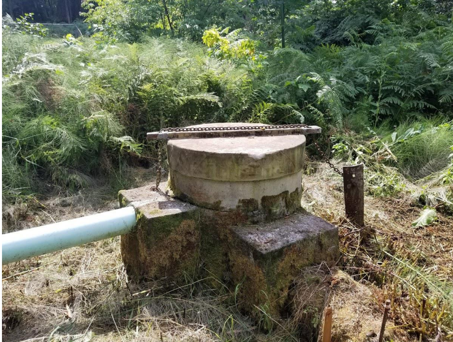
Left: Current collection system that needs replaced.
